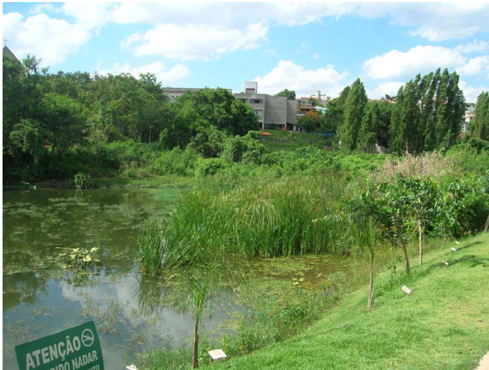
Figure 2. SUDS - Retention basin, Belo Horizonte
